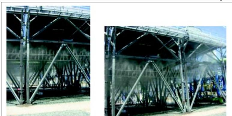
Figure 1 & 2. Illustration of proper chilling system where all the “fog” is evaporated before reaching the finned tube bundle on an induced draft air cooled heat exchanger unit.
